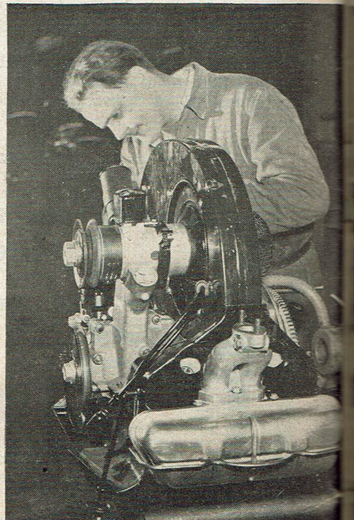
ONE MAN assembles each motor, initials it.
